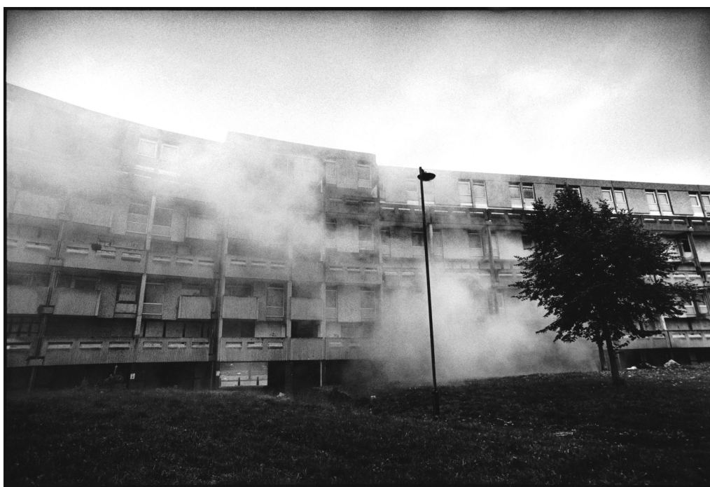
Figure 5 : Hulme Crescent in mist (Source: Sacha Lehrfreund, 1991).
