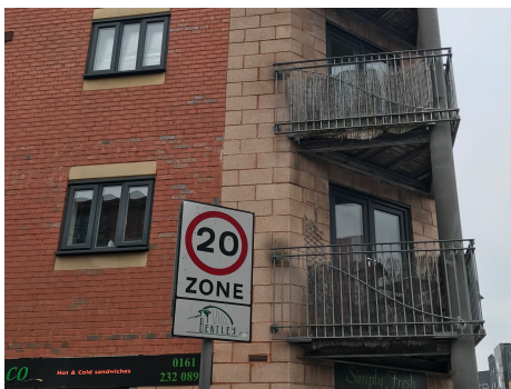
Figure 9: Private balconies along Stretford Road.
