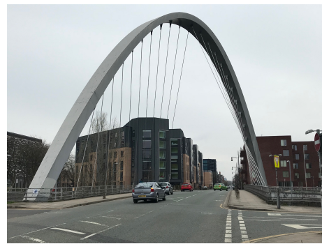
Figure 10: Hulme Arch, marking the entrance into Hulme.
